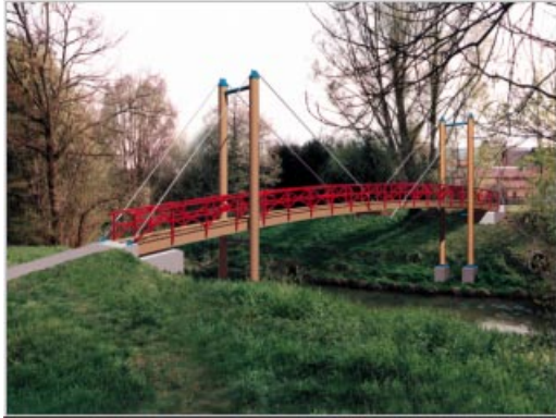
A CINEMA 4D object (the bridge) fits neatly into both a foreground and a background image (scene: Joachim Hoff)
